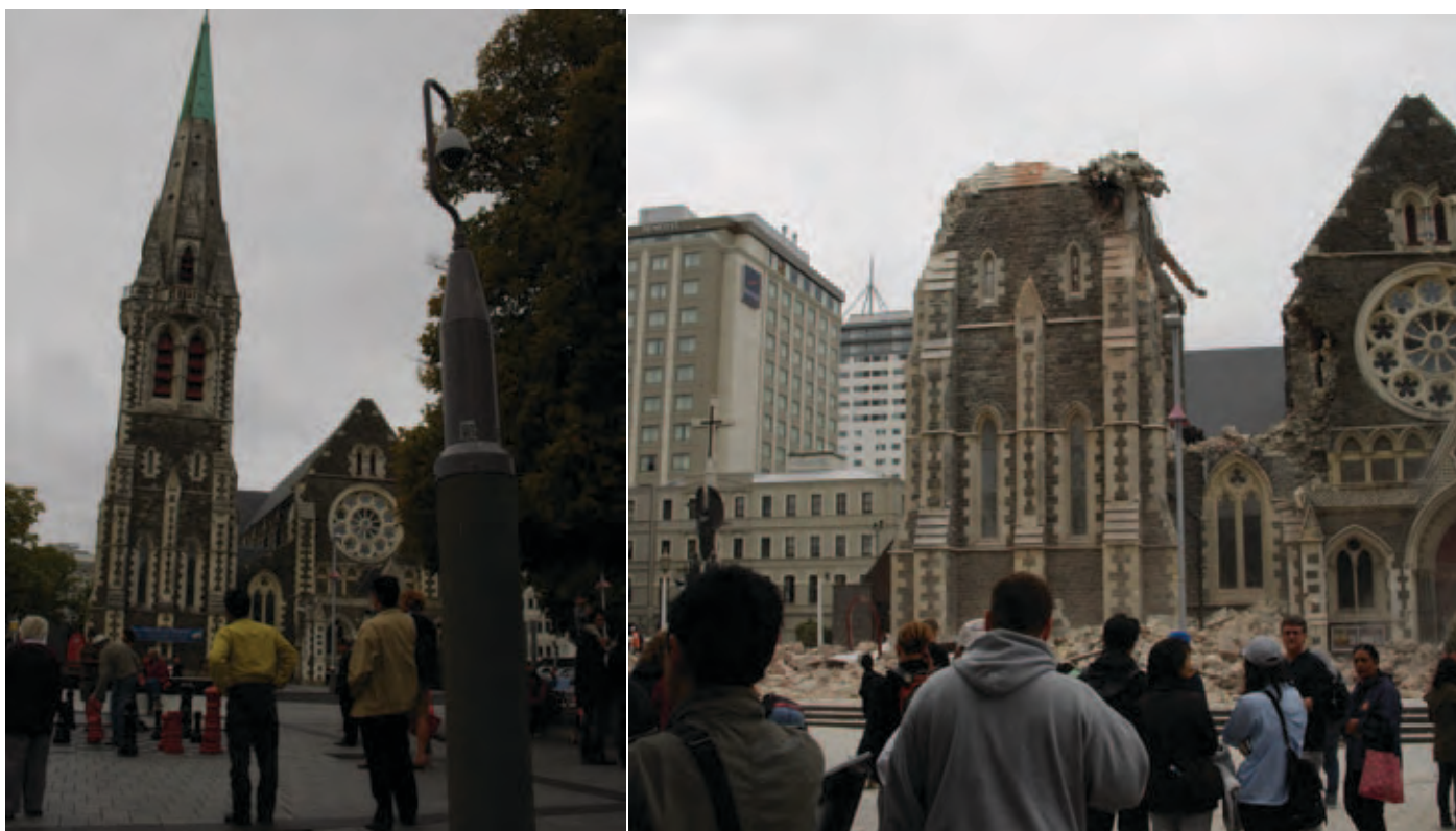
Christchurch Catholic Cathedral before and shortly after the earthquake on February 22, 2011
